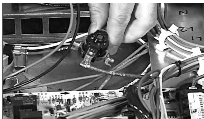
Figure 4-12. Limit Switch Removal.
