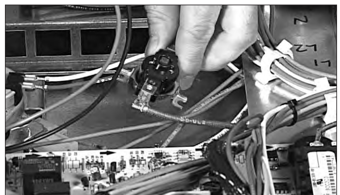
Figure 4-12. Limit Switch Removal.
