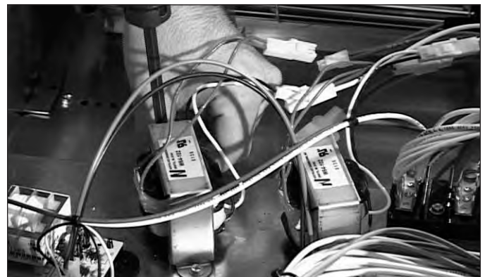
Figure 4-18. Light Transformer Removal.
