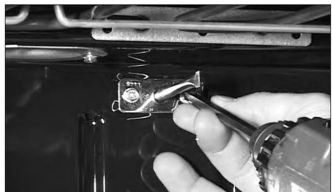
Figure 4-29. Temperature Sensor Removal.
