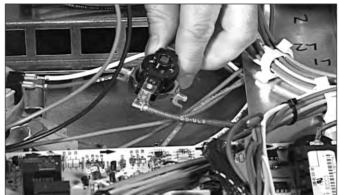
Figure 4-12. Limit Switch Removal.
